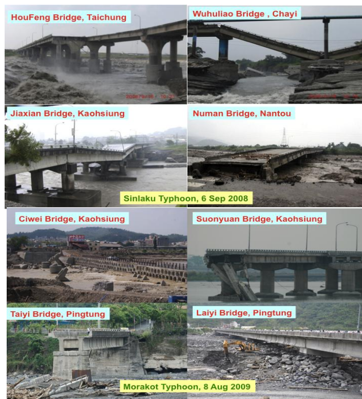
Fig. 1 Bridges failure during typhoon flood scour in Taiwan
