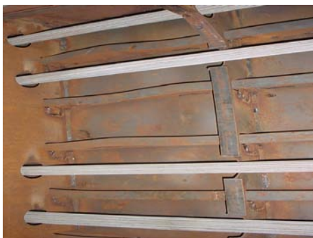
Figure 3 Local buckling mode in the test
