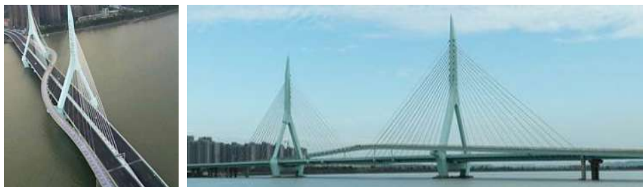
Figure 2.1 General view of the Mianyang First Bridge
