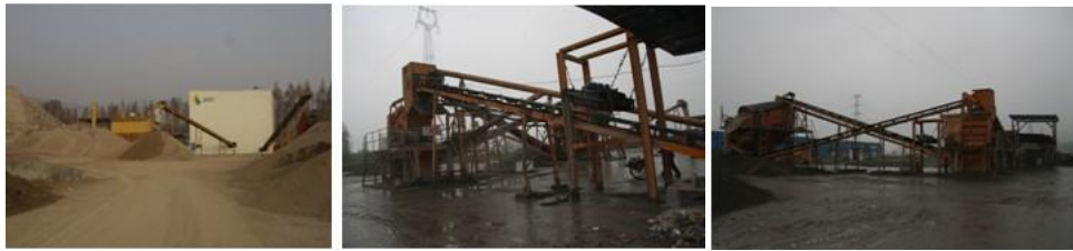
Fig. 2 Photographs of the recycling facility
