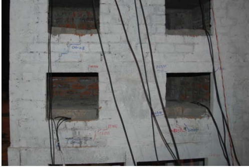
Figure 5.4 Cracks on spandrel wall of model H
