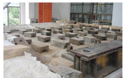
Figure 2.4 Water stains of frame 1
